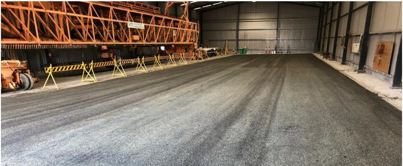
Figure 4.2 Test pavement after application of sprayed seal
