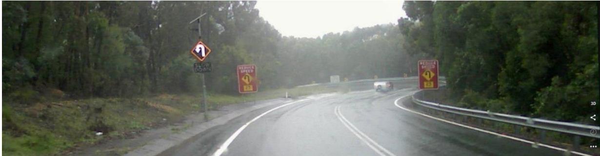
Figure 2.11: Road image of very tight radius turn on Kings Hwy (example 5)
